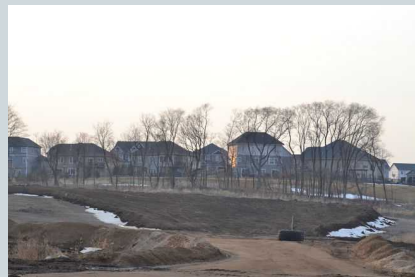
Looking into the remnants of the Upper Arboretum from Highway 19, where some completed homes already have new residents
